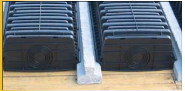
a travetti prefabbricati in c.a.p.
